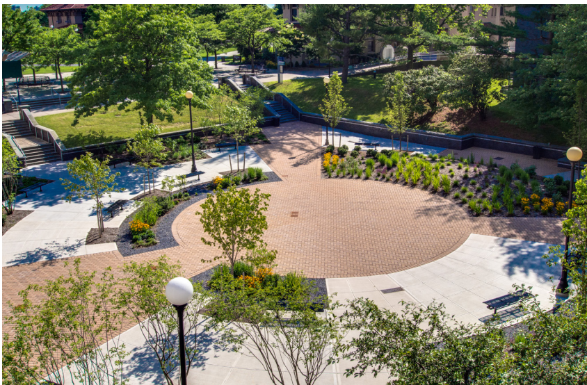
Kiely Hall - Permeable pavers and rain gardens, entrance plaza
