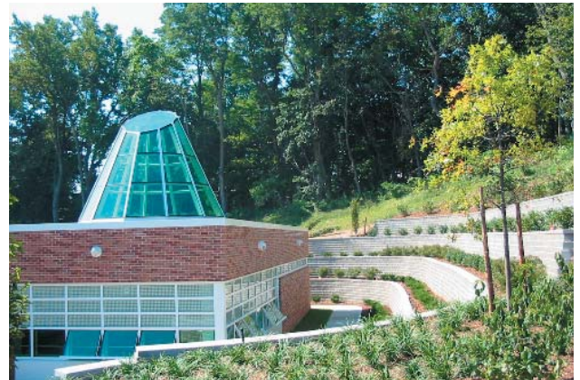
Salem Elementary School, Port Washington, NY
