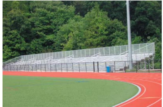
Greenwich High School Bleachers, Greenwich, CT
